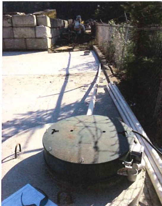
Picture 2 – looking east and oil water separator installed
